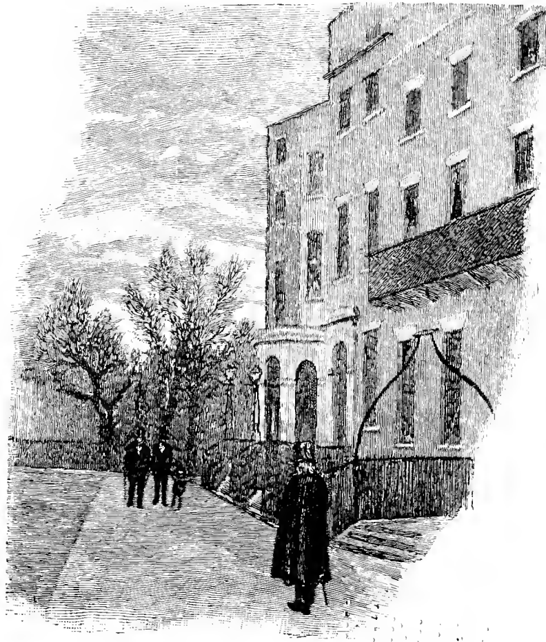
RUSSELL SQUARE, WHERE THE SEDLEYS BUILD
